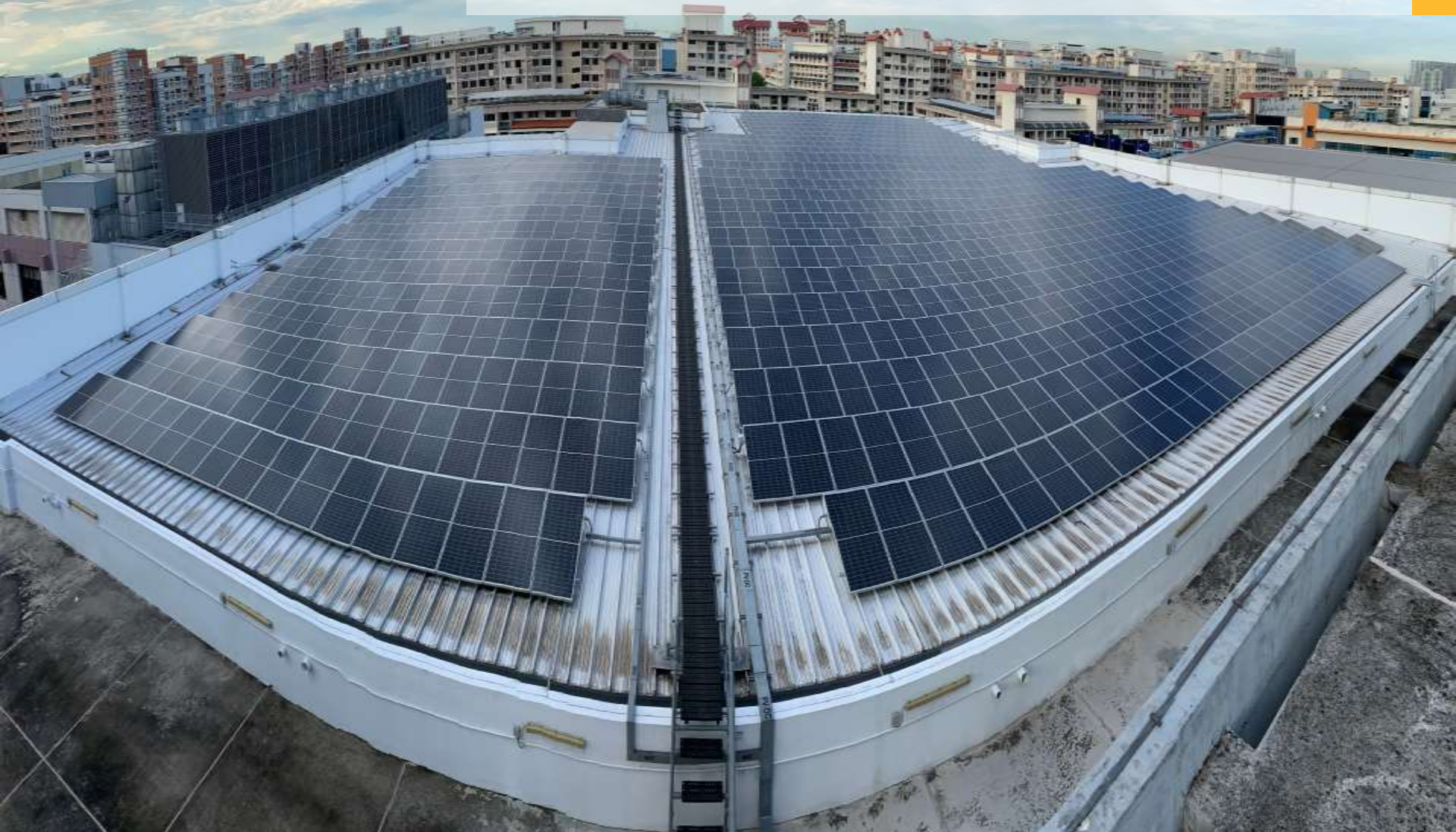
Solar Panels at the Rooftop of K&S Corporate Headquarters
