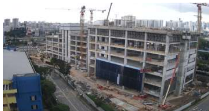
Completed Block 1 super structure and core walls; level 7 floor casting in Block 2; and level 2 casting in Block 3
